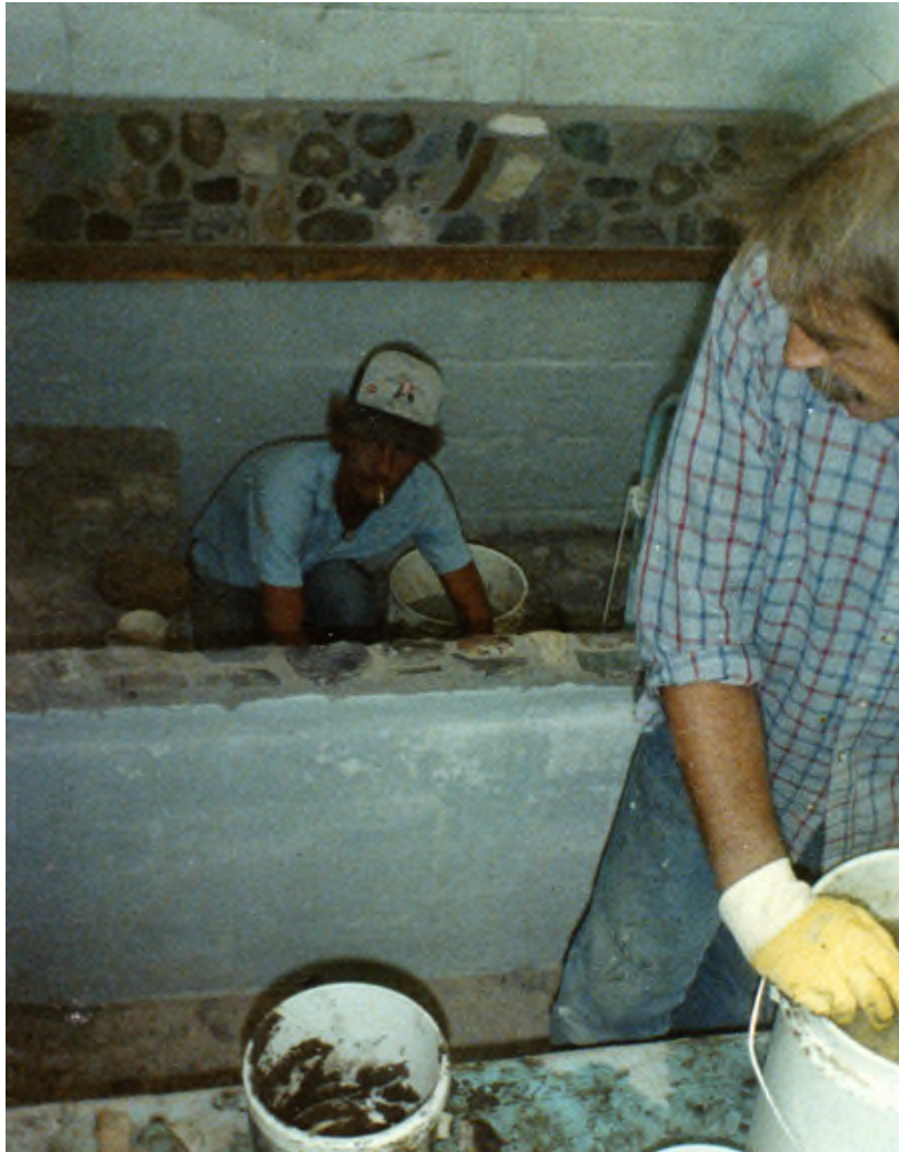
Finishing up the Indoor Hot Springs Pool
